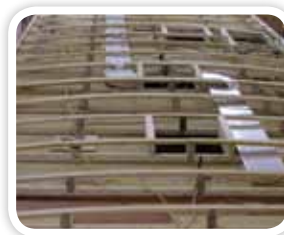
5" Roof truss with ducted AC and walkable decking
